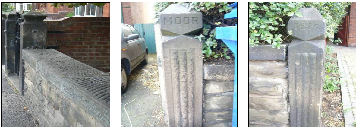
Tooled stone coping and gate piers with name inscriptions
