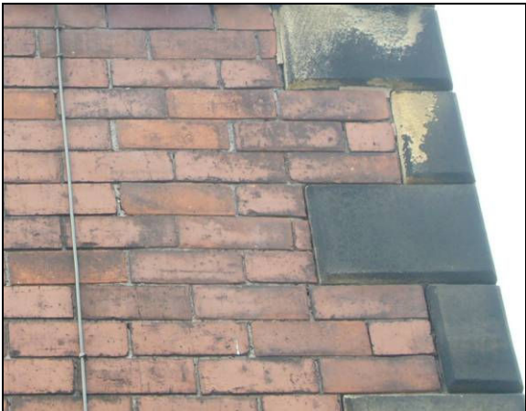
Stone quoins on brick wall
