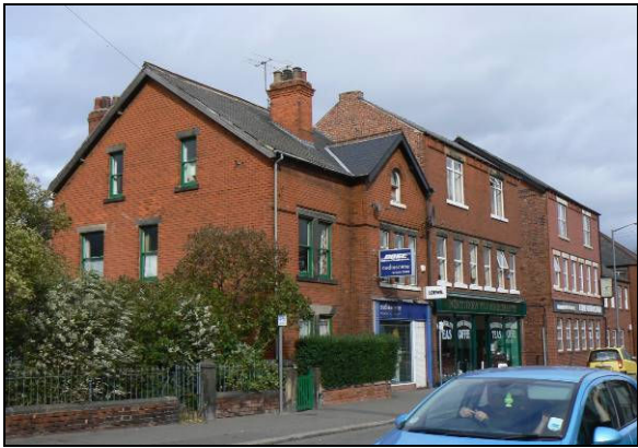
Red brick buildings
