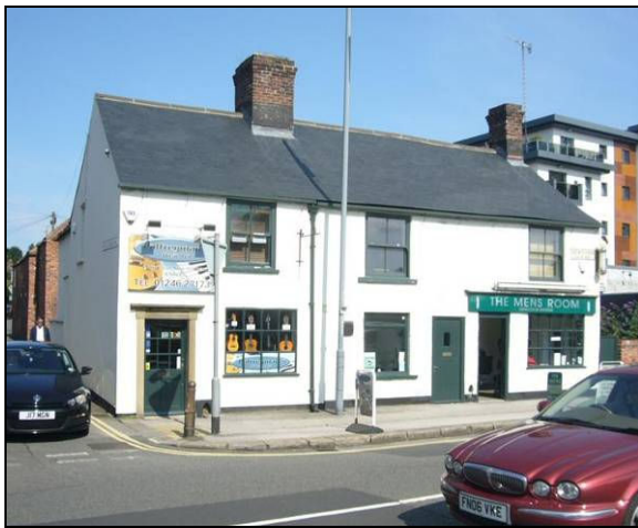
Nos. 169 & 171 Chatsworth Road
