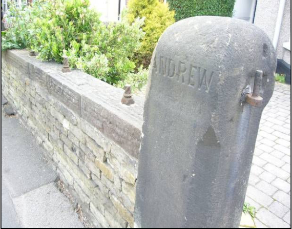
Remnants of iron railings on wall with tooled coping
